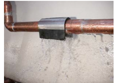
Loosen the bolt and separate the two parts of the clamp. Snap top half of clamp with rubber directly over leak
