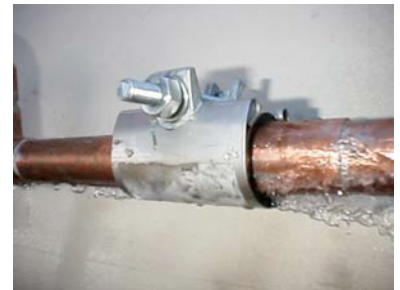
Spread open bottom section of clamp with nut facing out and slide on bottom half of clamp over top rubber section with arrows visible in the opening of bottom section.
